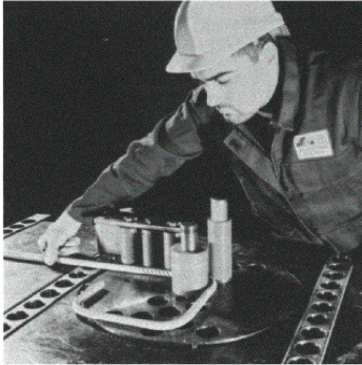
Figure 9.2(b) Bar bending in the factory. Acknowledgements to Allied Bar Coaters, Cardiff, Wales.
