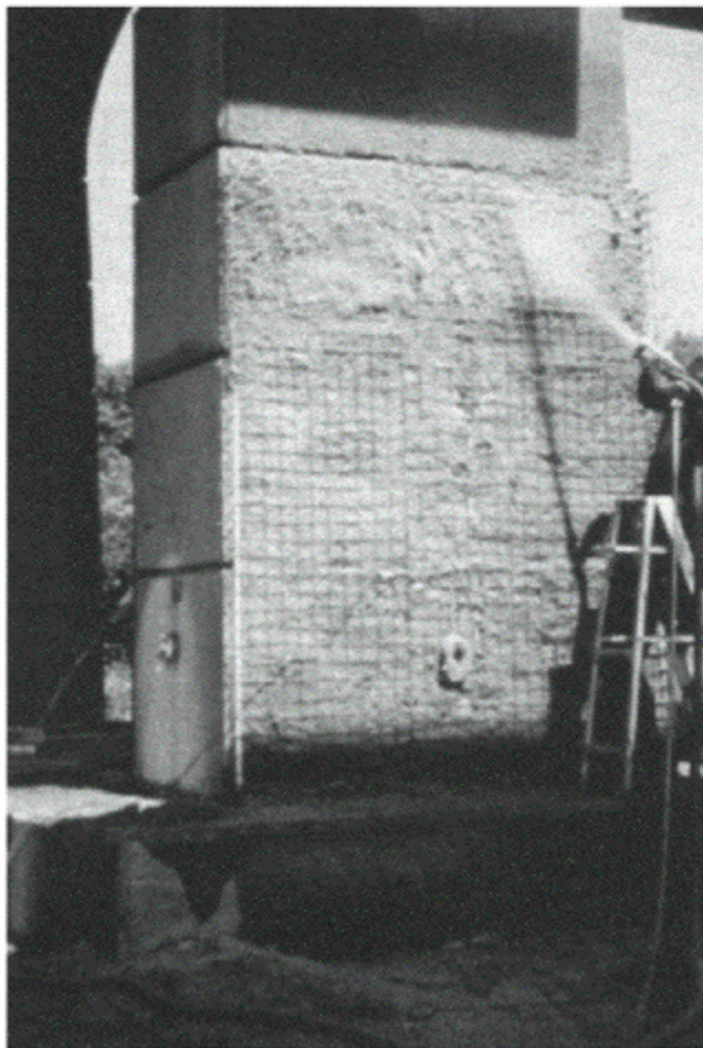
Figure 6.25 Desalination (electrochemical chloride extraction) trial: Burlington Skyway, Ontario, Canada 1989. Acknowledgements Ontario Ministry of Transportation, Eltech, SHRP.
