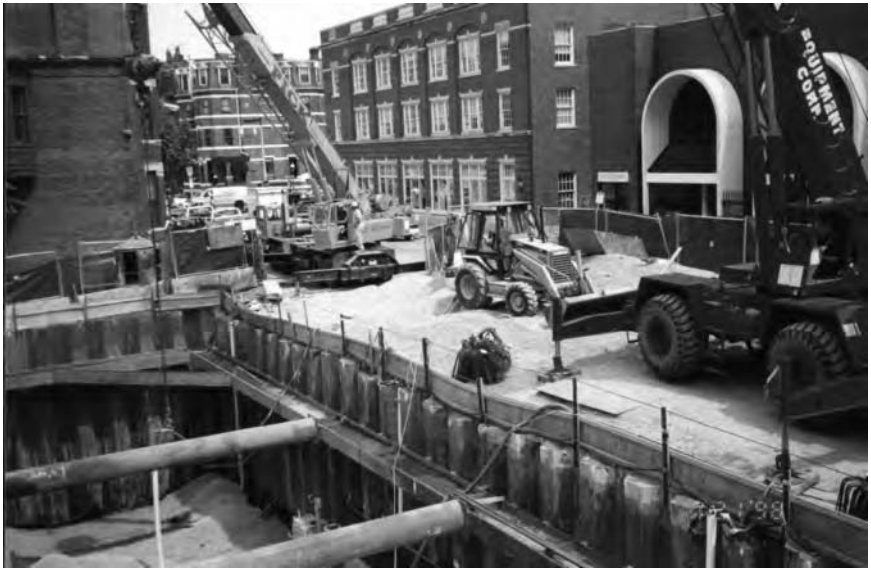
Figure 3.10 Overview of braced excavation, Boston, Massachusetts.
