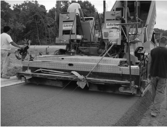
Figure 2.10 RCC pavement construction—Columbus, Ohio. (Photo by author.)
