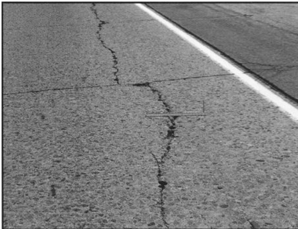
Figure 4.3 High severity longitudinal crack. (From Miller, J.S. and Bellinger, W.Y. 2003. Distress Identification Manual for the Long-Term Pavement Performance Program (Fourth Revised Edition) , FHWA-RD-03-031, p. 39. Washington, DC: Federal Highway Administration, United States Department of Transportation.)
