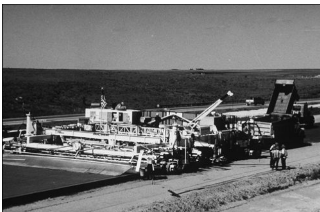
Figure 18.1 Slipform paving train. (Adapted from American Concrete Pavement Association (ACPA). 1996a. Construction of Portland Cement Concrete Pavements, Participant's Manual , FHWA HI-96-027, AASHTO/FHWA/INDUSTRY Joint Training, Washington, D.C.: Federal Highway Administration, United States Department of Transportation. Available on the web at http://isddc.dot.gov/OLPFiles/FHWA/014737.pdf : VI-6.)
