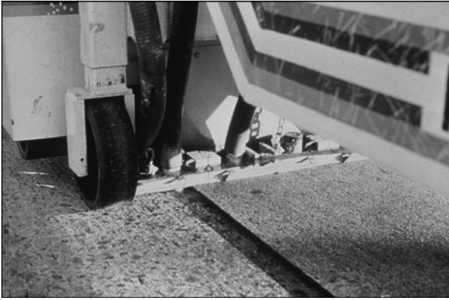
Figure 21.5 Diamond grinding. (From American Concrete Pavement Association (ACPA). 1996a. Construction of Portland Cement Concrete Pavements, Participant's Manual , FHWA HI-96-027, AASHTO/FHWA/INDUSTRY Joint Training, Washington, D.C.: Federal Highway Administration, United States Department of Transportation. Available on the web at http://isddc.dot.gov/OLPFiles/FHWA/014737.pdf : VIII-11.)
