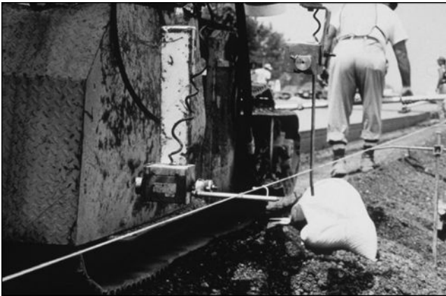
Figure 18.3 Stringline and paver sensing wand. (Adapted from American Concrete Pavement Association (ACPA). 1996a. Construction of Portland Cement Concrete Pavements, Participant's Manual , FHWA HI-96-027, AASHTO/FHWA/INDUSTRY Joint Training, Washington, D.C.: Federal Highway Administration, United States Department of Transportation. Available on the web at http://isddc.dot.gov/OLPFiles/FHWA/014737.pdf : VI-15.)
