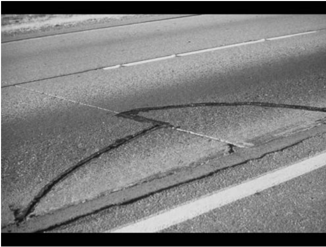
Figure 4.1 Corner breaks. (From American Concrete Pavement Association (ACPA) 1996a. Construction of Portland Cement Concrete Pavements, Participant's Manual, FHWA HI-96-027 , p. VIII-16. AASHTO/FHWA/INDUSTRY Joint Training, Washington, DC: Federal Highway Administration, United States Department of Transportation. Available on the web at http://isddc.dot.gov/OLPFiles/FHWA/014737.pdf .)
