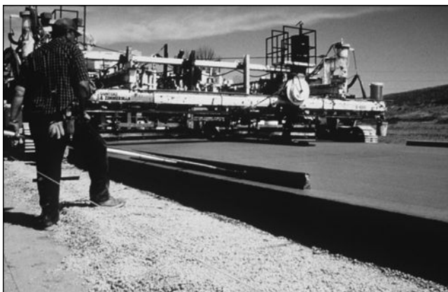
Figure 18.2 Concrete pavement produced by slipforming. (Adapted from American Concrete Pavement Association (ACPA). 1996a. Construction of Portland Cement Concrete Pavements, Participant's Manual , FHWA HI-96-027, AASHTO/FHWA/INDUSTRY Joint Training, Washington, D.C.: Federal Highway Administration, United States Department of Transportation. Available on the web at http://isddc.dot.gov/OLPFiles/FHWA/014737.pdf : VI-6.)
