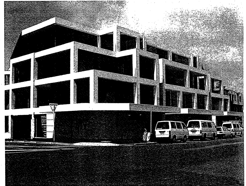
Photo 1.4 Typical reinforced concrete structure
