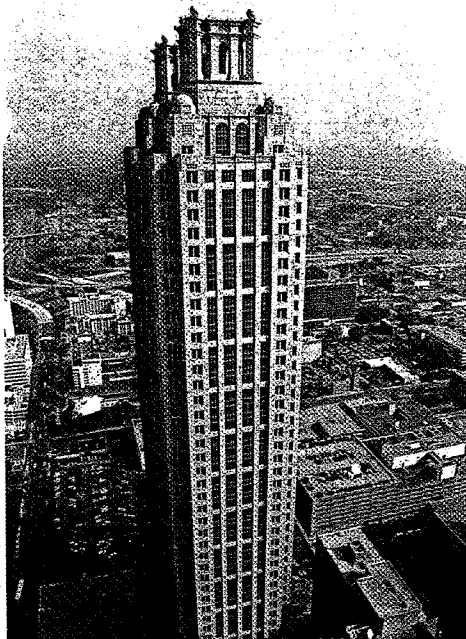
Photo 3.3 Peachtree Tower (1990), Atlanta USA (235m, 50 stories)
