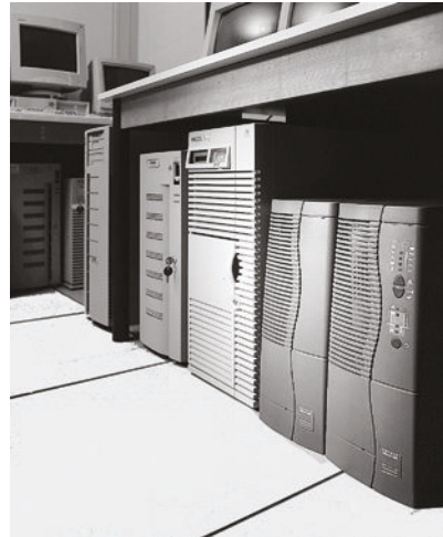
Fig. N32 UPS unit achieving disponibility and quality of computer system power supply
