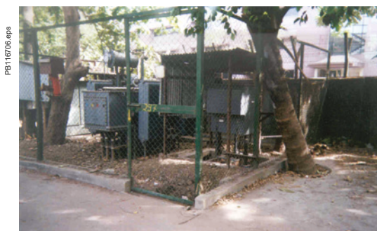
Fig. B53 Outdoor substation without enclosure
