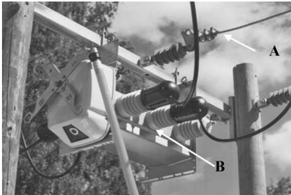
FIGURE 5.28 CT connections for pole-mounted switchgear.
