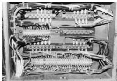
FIGURE 4-72B. Neatly installed bus bars and terminal strips. Note that everything is labeled, which will help in future troubleshooting. The four terminals stacked on one stud at the top left are acceptable under ABYC recommendations but would have been better spread out over a couple of studs. In the lower left the cable sheath reads “Boat Cable”—this is tinned, multistranded UL 1426 cable. A spare bus bar (middle right) has been fitted for future needs.
