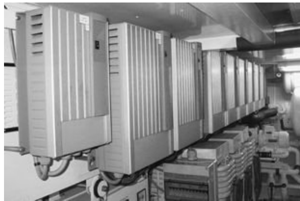
FIGURE 2-18. Cascaded battery chargers and DC-to-AC inverters on a superyacht, with multiple chilled-water air-conditioning condensing units beneath them. ( Courtesy Mastervolt )
