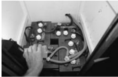
FIGURE 3-2A. Topping off wet-cell batteries. In order to maintain wet-cells, it is essential to have good access.
