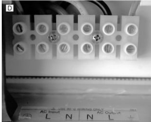
FIGURE 6-29D. A typical AC wiring box on an inverter with an automatic transfer switch.
