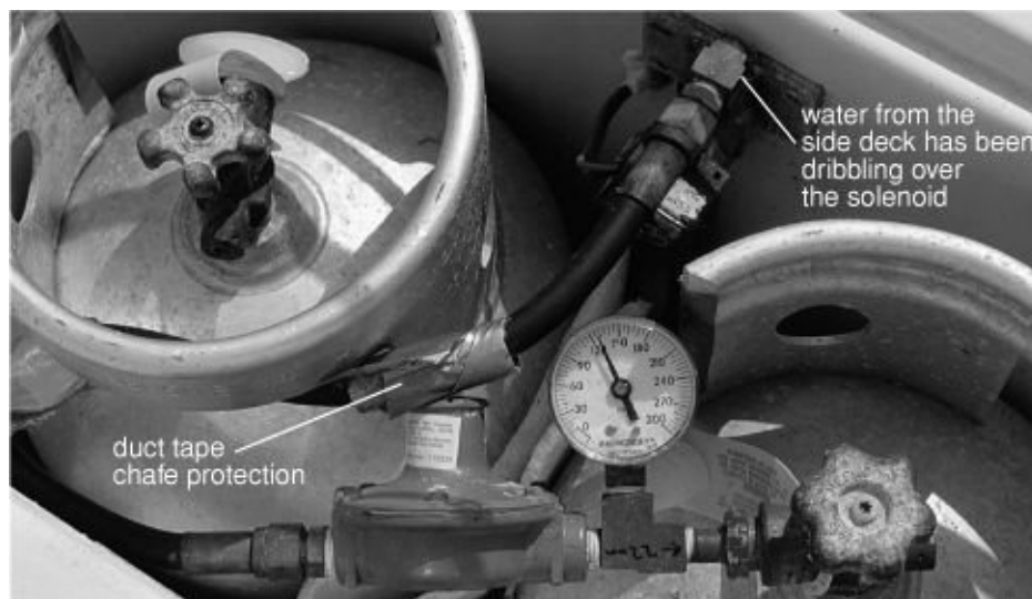
FIGURE 15-6B (below). A common two-cylinder installation without a selector valve. To change cylinders, the regulator must be moved from one cylinder to the other. These are old-style (non-OPD)
