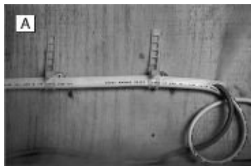
FIGURE 4-74. How a short circuit occurs.
