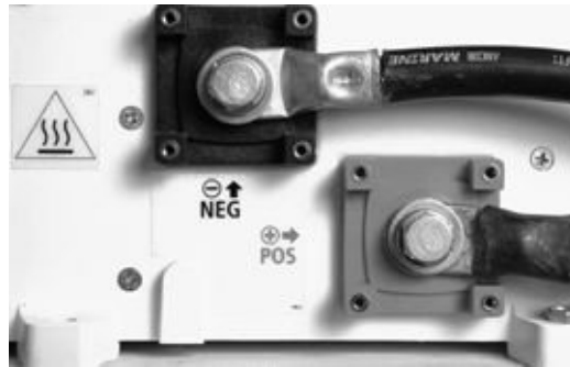
FIGURE 6-27. DC cable installation on an inverter. Note the heavy cables and bolted connections, which will now be covered by protective boots.
