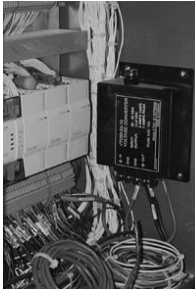
FIGURE 2-12. A DC-to-DC converter supplying a stable, filtered voltage to sensitive equipment. ( Analytic Systems )
