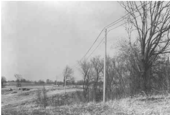
FIGURE 2.35 A typical 12.47 kV line with a single circuit and wood pole. It has a newer type of pole-top construction. (Union Electric Company.)
