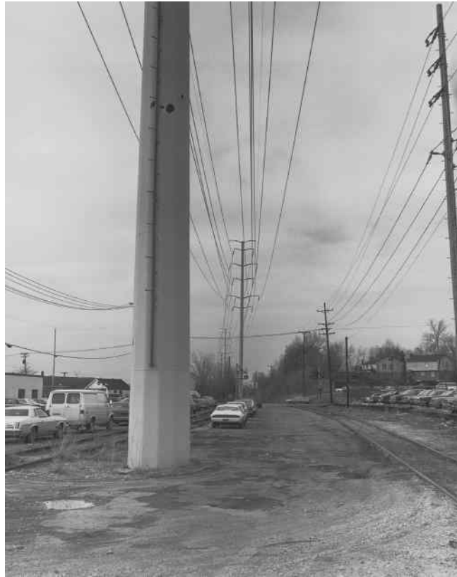
FIGURE 2.6 A double-circuit 138 kV line built by using steel poles, having two 138 kV circuits underbuilt. (Union Electric Company.)
