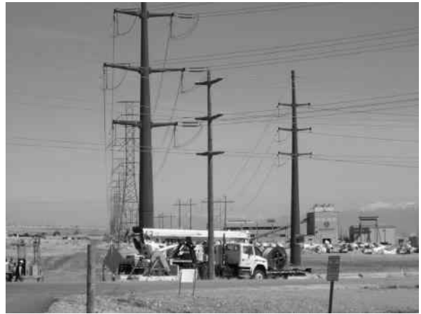
FIGURE 2.21 A 115 kV transmission line and a 345 kV transmission line with corner towers. (Courtesy of West Power Inc.)
