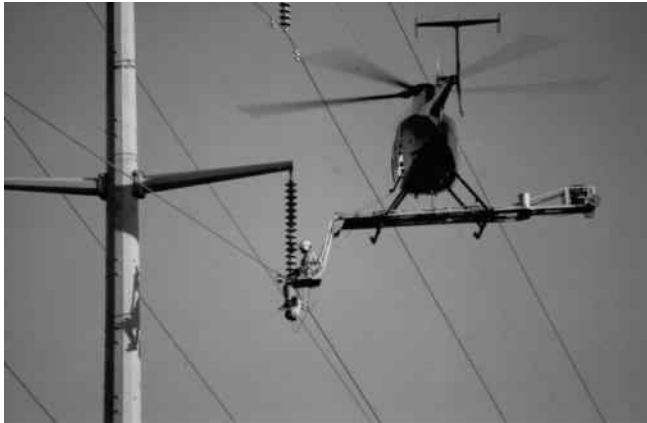
FIGURE 2.15 A lineman working from a helicopter platform.
