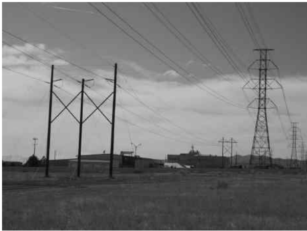
FIGURE 2.19 A 115 kV transmission line and a 230 kV transmission line side by side. (Courtesy of West Power Inc.)
