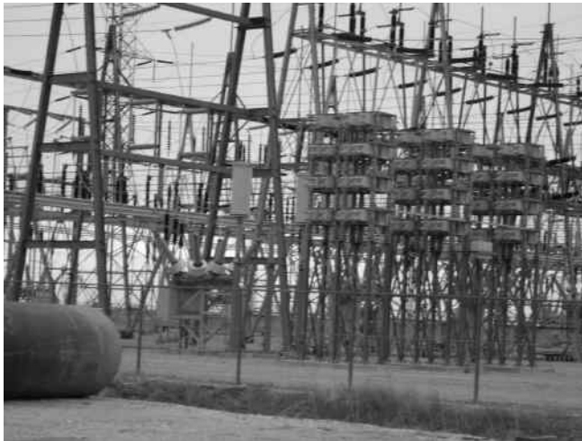
FIGURE 2.23 A 230 kV switchyard. (Courtesy of West Power Inc.)
