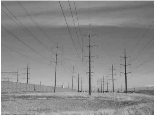
FIGURE 2.20 A cluster of four transmission lines side by side. (Courtesy of West Power Inc.)
