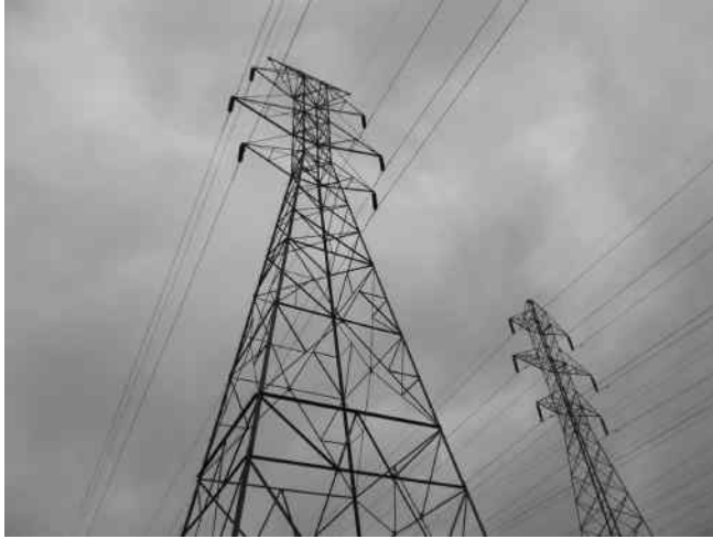
FIGURE 2.22 A 345 kV transmission line and a 115 kV transmission line side by side. (Courtesy of West Power Inc.)
