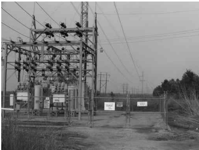
FIGURE 2.18 A 230/161 kV substation with a 230 kV transmission line passing by. (Courtesy of West Power Inc.)
