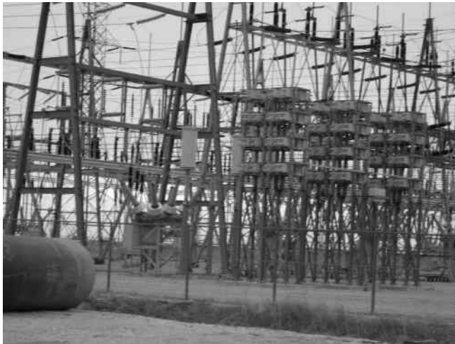
FIGURE 2.25 A 230/34.5 kV switchyard. (Courtesy of West Power Inc.)
