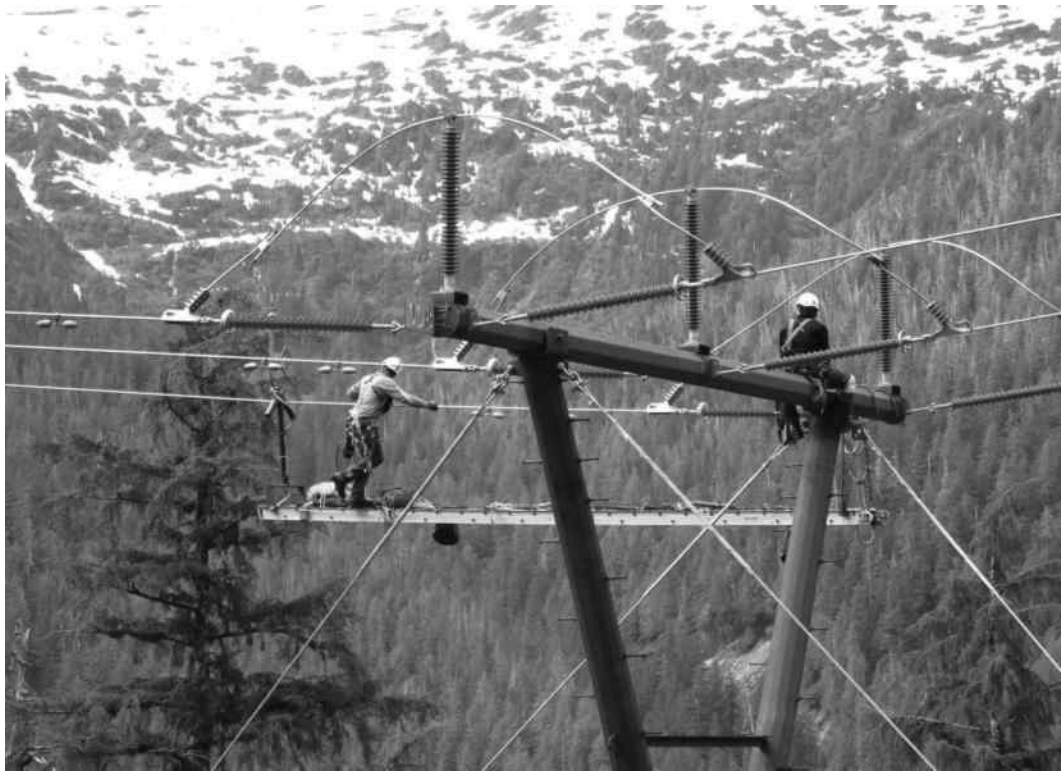
FIGURE 13.22 A crew is working on pole-top construction.
