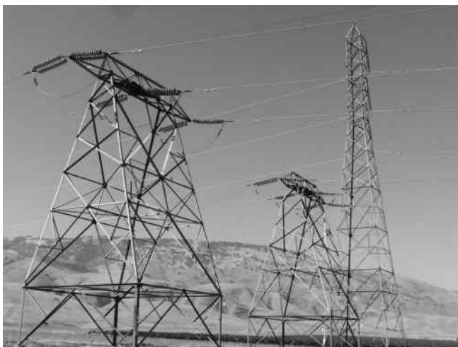
FIGURE 2.16 Two 345 and 230 kV transmission lines side by side. (Courtesy of West Power Inc.)
