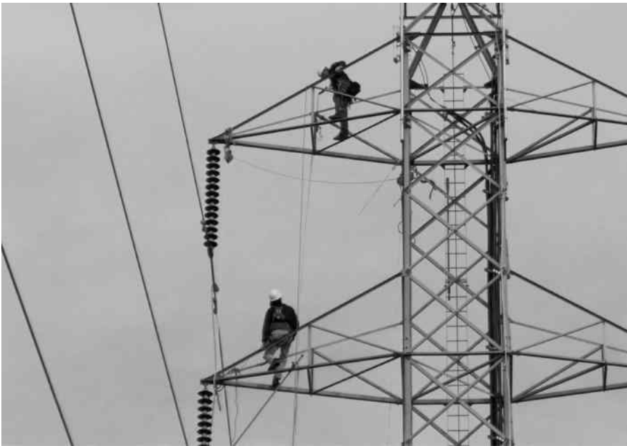
FIGURE 1.4 A transmission line is being upgraded.
