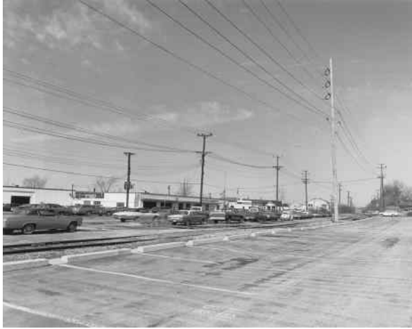
FIGURE 2.34 A typical 34.5 kV line with a double circuit and wood poles. It also has a 4.16 kV underbuilt line and a 34.5 kV switch. (Union Electric Company.)
