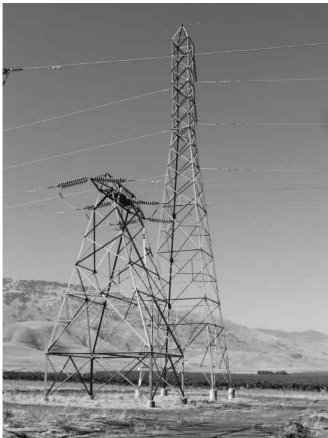
FIGURE 2.17 A 345 kV transmission line and a 230 kV transmission line side by side. (Courtesy of West Power Inc.)
