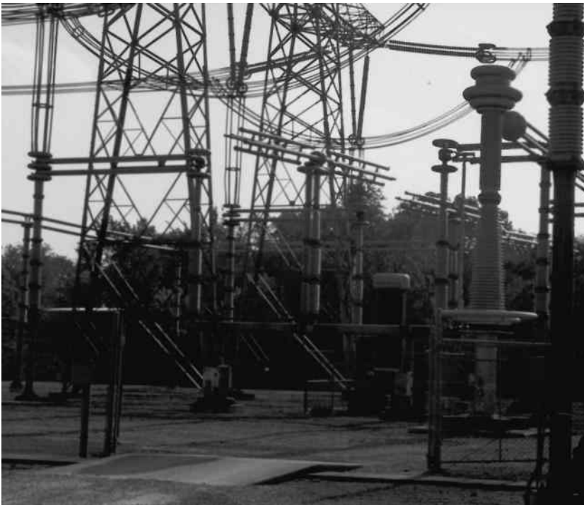
FIGURE 6.11 An 800 kV disconnect switch on the ac side at the same converter station.
