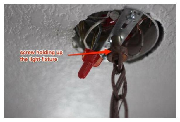
Same image as above, this one pointing out how to remove the light fixture. Once the wires are disconnected, unscrew here and the fixture is off the ceiling. Again, this may vary given the light fixture you're working with.
