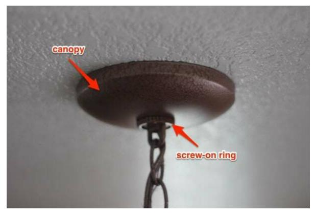
The fixture I was replacing used a simple screw-on ring to hold up the canopy (and fixture). Each fixture is different, but no matter what it is, it should be pretty easy to figure out.
