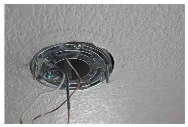
New baseplate. The two screws holding it up to the ceiling are a universal distance apart. You can also see the green ground screw (more on that below).
