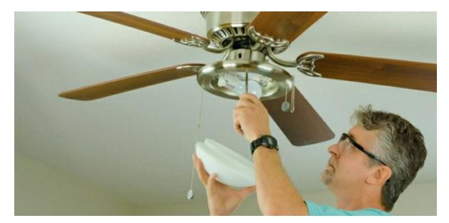
Once you discover that your switch is working, move to checking the ceiling fan wiring. Again, turn off the electricity to the room at the breaker box and, if you have someone to hold up the ceiling fan while you work, then just unscrew it from the ceiling. If you don't have an assistant, you will need to remove the fan blades and then unscrew the ceiling fan from its mounting bracket.
