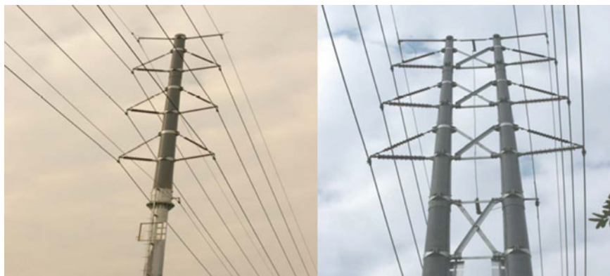
Fig. 2.6 A composite tower for 110 kV overhead lines in China with a single pole (left); with double poles (right) [45]
