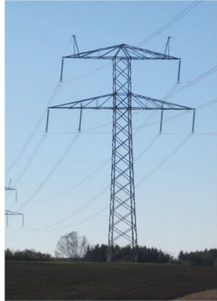
Fig. 1.2 a A prototype of new pylon for 400 kV overhead line between Aalborg and Aarhus (in Denmark), b A conventional Donau pylon for 400 kV overhead line [14]
