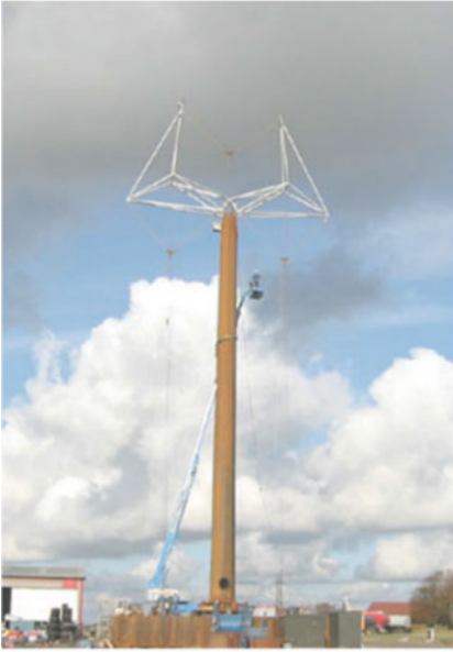
Fig. 1.2 a A prototype of new pylon for 400 kV overhead line between Aalborg and Aarhus (in Denmark), b A conventional Donau pylon for 400 kV overhead line [14]
