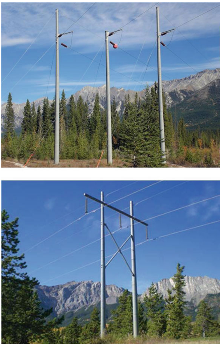
Fig. 2.7 Commercialized Fiber Reinforced Plastic (FRP) towers in transmission lines manufactured by RS Technologies Inc., Canada [46]
