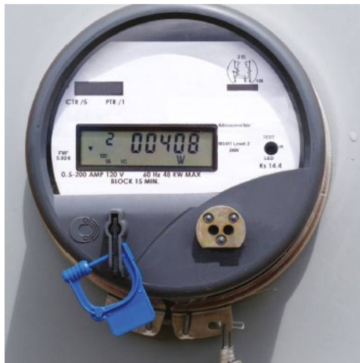
Figure 3.14 An example of a smart electricity meter.
