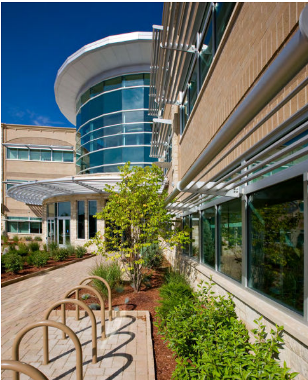
ILI's products, like this sunshade, help reduce energy loads. Attention to human health is new. Courtesy: Industrial Louvers, Inc.
