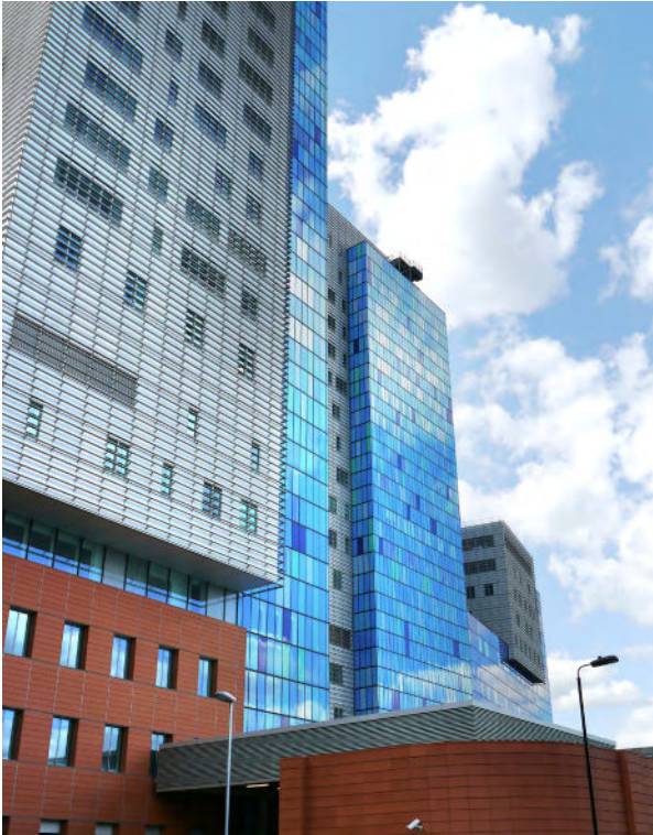
The facade manufacturer for the Royal London Hospital removed cadmium from the panel formulation.
