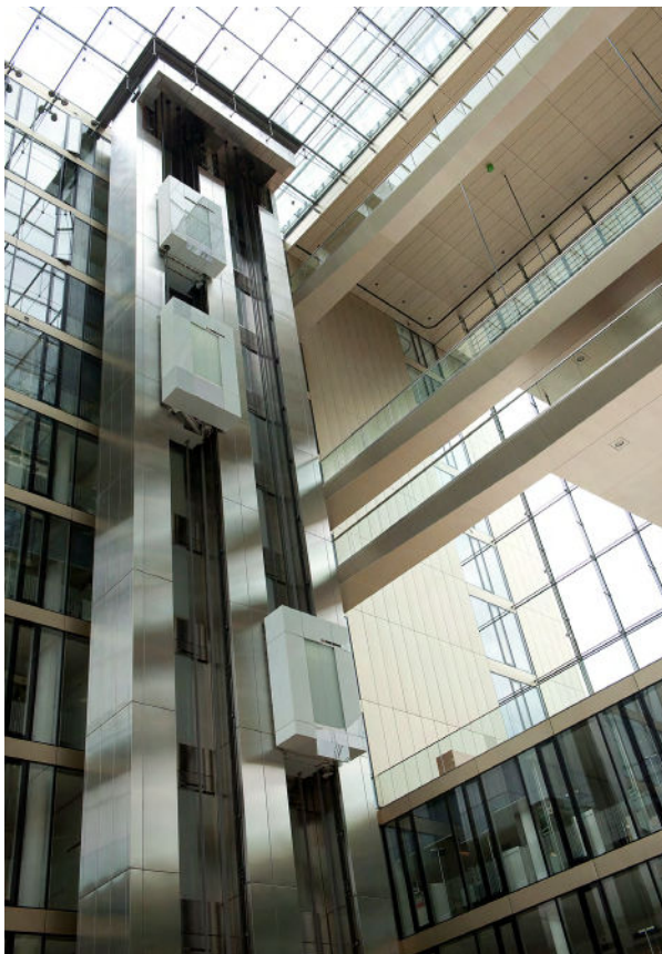
Two elevator cabs travel independently—one above the other in the same shaft.
