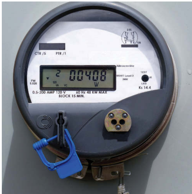
Figure 3.14 An example of a smart electricity meter.
