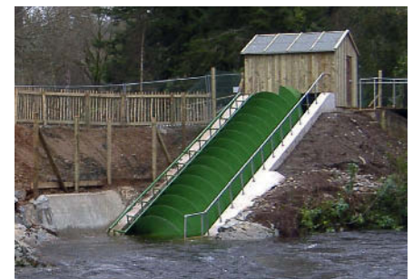
Figure 3.24 An example of an Archimedian Screw at the River Dart country park, Devon. Credit: WRE Limited.
