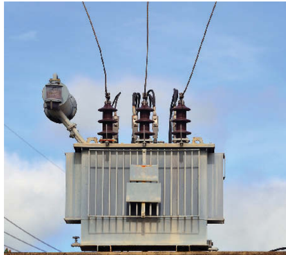
Figure 2.56 A 3ph transformer.
