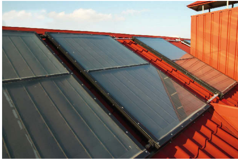
Figure 3.17 Solar hot water panel.
