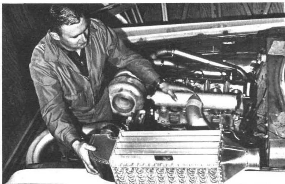
"Turbo Honker" Dodge with 7:1 compression ratio hemi engine assembled by Bud Faubel and George Weiler in 1966. Two ice-water-cooled intercoolers, one in each front fender and two T18 free-floating AiResearch turbos were used. Car turned 160 MPH in the quarter mile. Alex Walordy photo.
