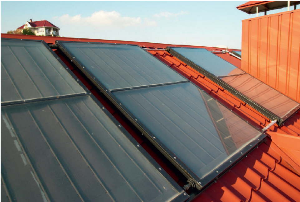
Figure 2.3 Photo of a solar hot water panel.
