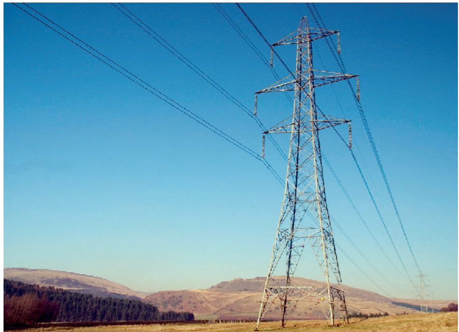
Figure 4.5 Transmission line steel pylon.
