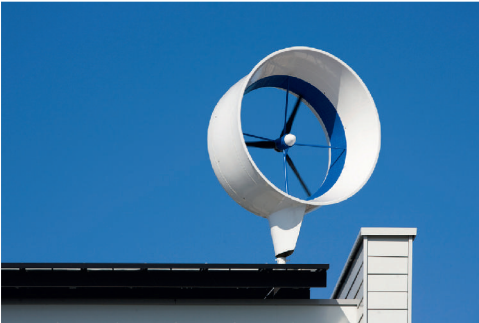
Figure 2.5 Small wind generator on a domestic property.
